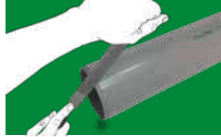
6. Solvent Cement application
